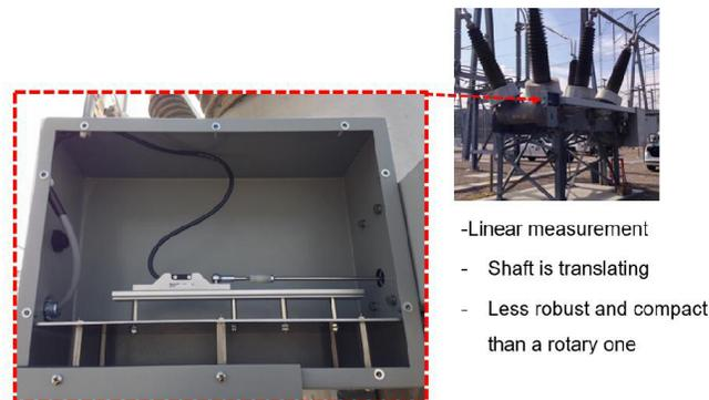
**Figure 10 - Linear transducer with linkage**
